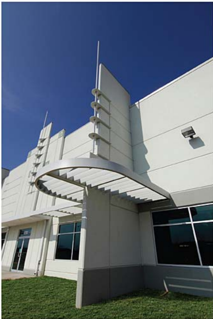
ABOVE, BELOW: Heavy Fleet Corp. Headquarters in Manassas, Va., was another of the Tilt-Up Concrete Assn.'s 2008 Tilt-Up Achievement Award winners. With the objective of constructing a "South Beach" art deco warehouse and distribution center in an industrial park for Heavy Fleet, tilt-up concrete provided the ideal solution. Vertical fins and spires were used to break-up the façade and provide an interesting elevation. Horizontal elements include a painted steel sunscreen/canopy and horizontal reveals. Pineapple Grove precast medallions were applied in recessed areas above the main entrance to architecturally enhance the panels.
