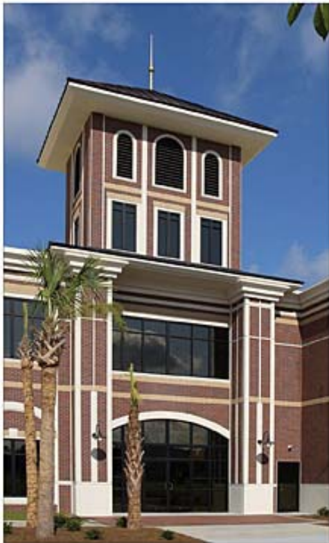
RIGHT: American LaFrance's Office and Warehouse Facility in Summerville, S.C. earned a 2008 Tilt-Up Achievement Award from TCA, in part for its two 51-ft.-tall brick inlay panels, connected by two spandrel panels at the top and eight accent panels at the base.
