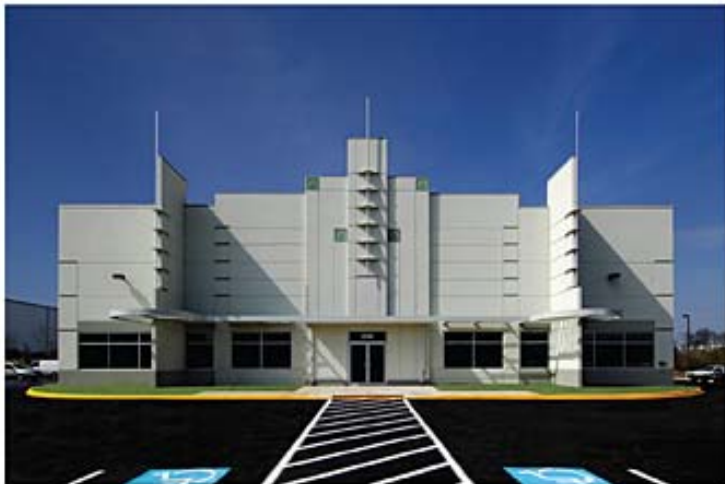
ABOVE, BELOW: Heavy Fleet Corp. Headquarters in Manassas, Va., was another of the Tilt-Up Concrete Assn.'s 2008 Tilt-Up Achievement Award winners. With the objective of constructing a "South Beach" art deco warehouse and distribution center in an industrial park for Heavy Fleet, tilt-up concrete provided the ideal solution. Vertical fins and spires were used to break-up the façade and provide an interesting elevation. Horizontal elements include a painted steel sunscreen/canopy and horizontal reveals. Pineapple Grove precast medallions were applied in recessed areas above the main entrance to architecturally enhance the panels.
