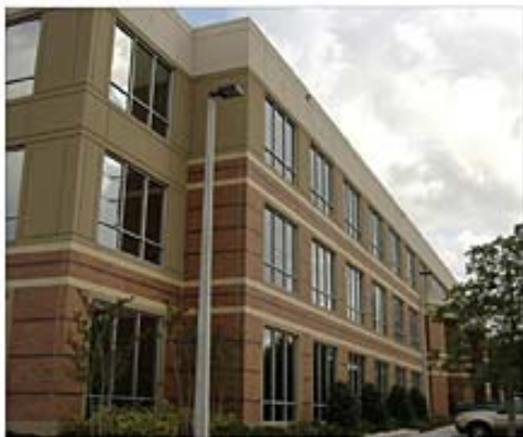
RIGHT: Highland Oaks 5, a 101,955-sq.-ft. office facility in Tampa, Fla., was another of TCA's 2008 Tilt-Up Achievement Award winners. Tilt-up panels were used to achieve a brick deco look that was durable and economical.
