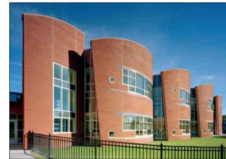
Best Contemporary Design Project - Brick John S. Martinez Elementary School New Haven, Connecticut Architect: Svigals + Partners, LLP Mason Contractor: B.W. Dexter II, Inc. Owner: City of New Haven CM: Fusco Corporation Engineer: Michael Horton Associates, Inc. Photography: Woodruff/Brown
