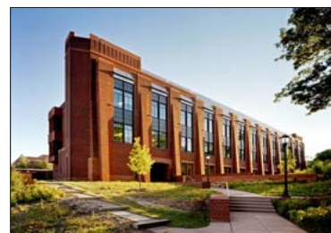
Educational Category - College Classrooms Yale Class of 1954 Chemistry Research Building New Haven, Connecticut Architect: Bohlin Cywinski Jackson Mason Contractor: NER Construction Management CM: William A. Berry & Son Owner: Yale University Engineer: Cannon Design Photography: Nic Lehoux Photography
