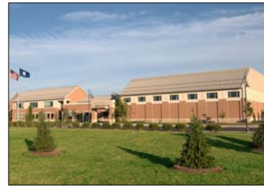
Educational Category - Elementary Schools Nayaug Elementary School Glastonbury, Connecticut Architect: Moser Pilon Nelson Architects Mason Contractor: Joe Capasso Mason Enterprises, Inc. CM: Industrial Construction Company Owner: Town of Glastonbury Engineer: Macchi Engineers, LLC Photography: Moser Pilon Nelson Architects
