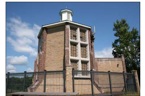
Commercial Category - Industrial Projects Fisher Meadows Well Pump House Avon, Connecticut Architect: Tuthill & Wells Architects Mason Contractor: John Filloramo Construction Company CM: Master's Construction Corporation Owner: Avon Water Company Engineer: Buck and Buck LLC, Engineers Photography: IMI
