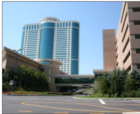
Special Award Project Foxwoods Casino MGM Grand Hotel Ledyard, Connecticut Architect: HKS, Inc Owner: Mashantucket Pequot Tribal Nation CM: Perini Building Company Engineer: Cagley Harman & Associates
