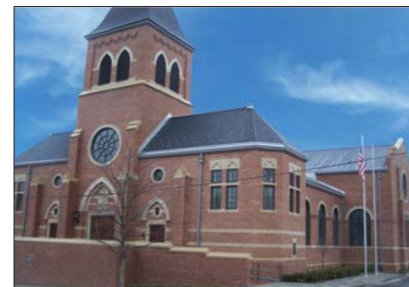
Institutional Category - Churches Sacred Heart Parish Church Weymouth, Massachusetts Architect: The S/L/A/M Collaborative Mason Contractor: Commercial Masonry Corporation Owner: Roman Catholic Archdiocese of Boston Engineer: The Collaborative Engineers Photography: The S/L/A/M Collaborative
