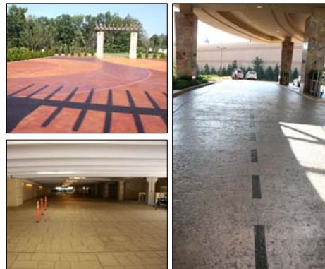
Special Award Project - Decorative Concrete Foxwoods Casino MGM Grand Hotel Ledyard, Connecticut J.L. Marshall & Sons, Inc.
