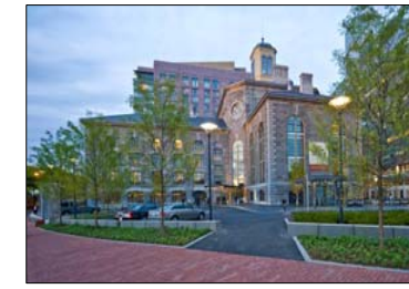
Restoration Category - Large Projects The Liberty Hotel Boston, Massachusetts Architects: Cambridge Seven Associates, Inc. Mason Contractor: Phoenix Bay State CM: Weidlinger Associates, Inc. Owner: Carpenter & Company, Inc. Photography: Cambridge Seven Associates, Inc. / Peter Vanderwarker / Michael Weschler Photography
