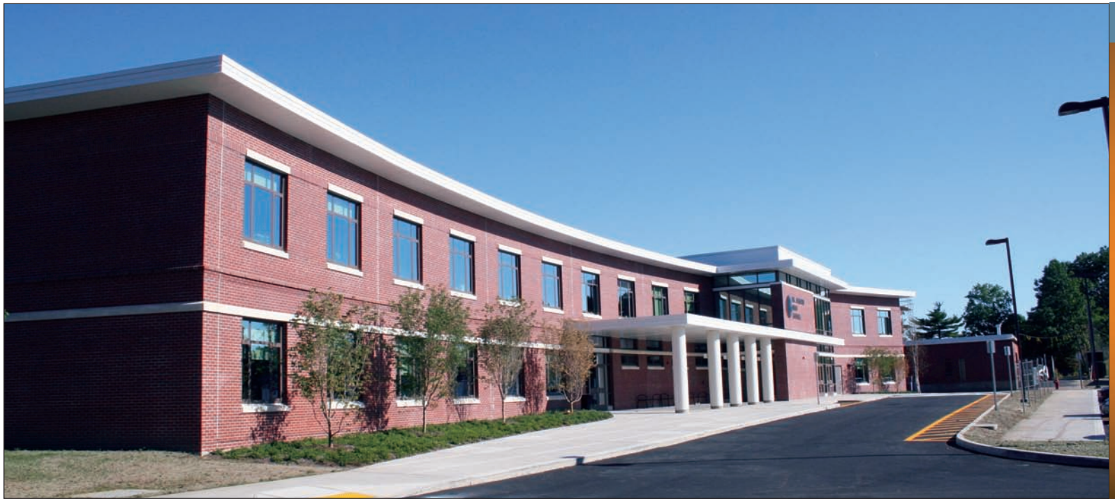
Also pictured on page 30, Manchester High School in Connecticut showcases modern masonry cavity wall construction. Material selection is crucial in ensuring a moisture management system that achieves the desired performance.
